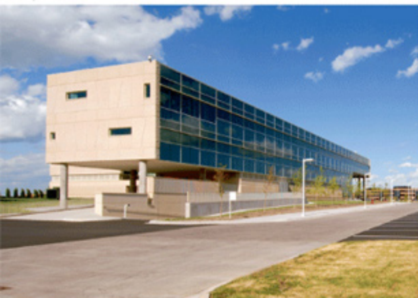
The building form was established to enhance natural light and views to the outside. East-to-west building orientation and narrow floor plates provide effective daylighting. Photo: Lucie Marusin
